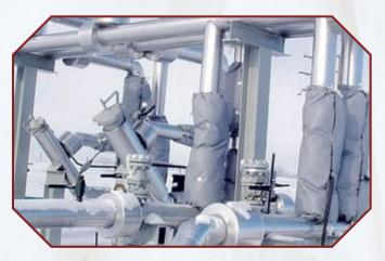
The cold insulation work comprises between temperatures - 200°C to 20°C. The vessels and pipelines to be insulated will be cleaned so as to make the same free from dust and grease. These vessels and pipelines will be applied with bituminous coating and insulation of Thermocol / PUF will be fixed with bitumen compound.
